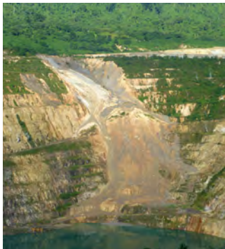
Figure 2 - 150m+ high gully on mine pit slope formed through rainfall-induced landslides over 5 year period. Deteriorating, clay-altered mass and relic geologic structures.
