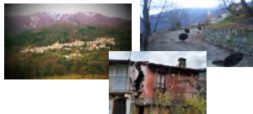
General View of the Site
