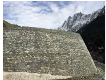
Protective Reinforced Earth® wall, Zmorth Project (India)
