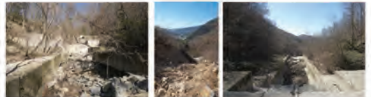
Damages in the stabilization structures realized after the 1970 event
