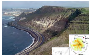
Cracks at the coronation and the cliff side (1985-today)
