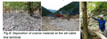
Fig.8: Deposition of coarse material at the ski cable line terminal
